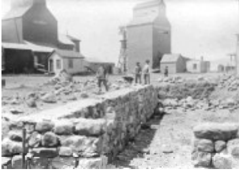
The stone foundation being laid in May 1908
