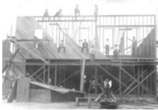
The impressive structure under construction
