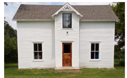
The Solheim House sporting its newly restored exterior
