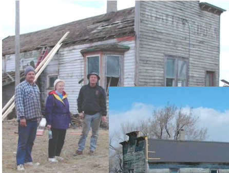
David and Charles Bolin and owner Audrey Solheim during roofing project in April.
