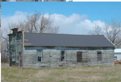
New steel roof on the service station and facial repaired.
