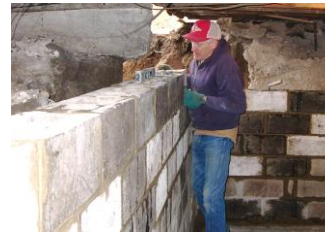
Paul Gunderson, volunteer contractor
