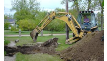
Mark Faul with his backhoe at the Melby-Rogness House
