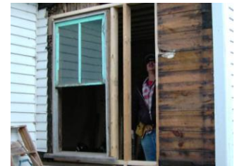
Perry Anderson restored water damaged portion of dining room wall
