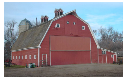
Oldest known hip-roof barn built in 1910 for homesteader Ole J. Rodne. Builder unknown. Present farm of Bill Ongstad. Notice wooden cupolas.
