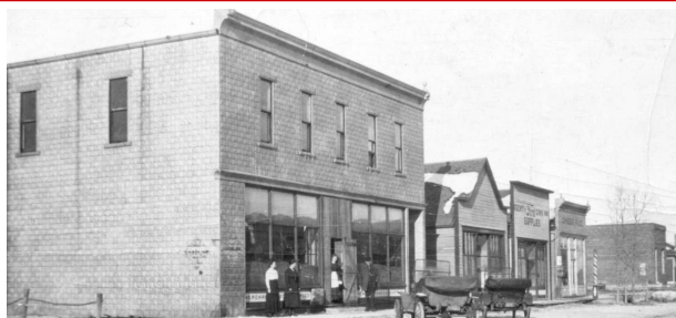
During 1920-1926, Fagerlund Lodge met in the upstairs ballroom of the C.C. Melby Store (foreground). Photo provided by Myrtle Sailer.
