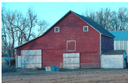
Gable-roof barn built in 1909 by homesteader, Jacob Seltvedt with the help of his neighbors. Present farm of his grandson, Don Seltvedt.
