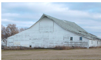
Gable-roof barn built in the 1890s for/by homesteader, Ole L. Rodne. Present farm of his son, Berger Rodne.
