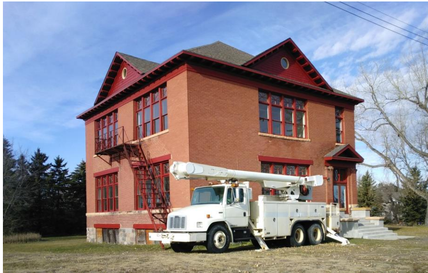
Manfred School – painting of east dormer in progress using a lift truck, Nov. 2021
