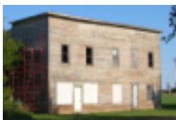
Hotel structure was stabilized by June 2007. Exterior now under restoration.
