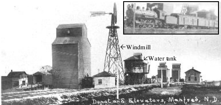
Water from the James River was pumped by windmill to the water tank for use in supplying water to the steam-powered locomotives
