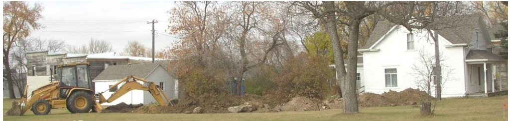
Digging the trench for the water line on south side of the Melby-Rogness House
